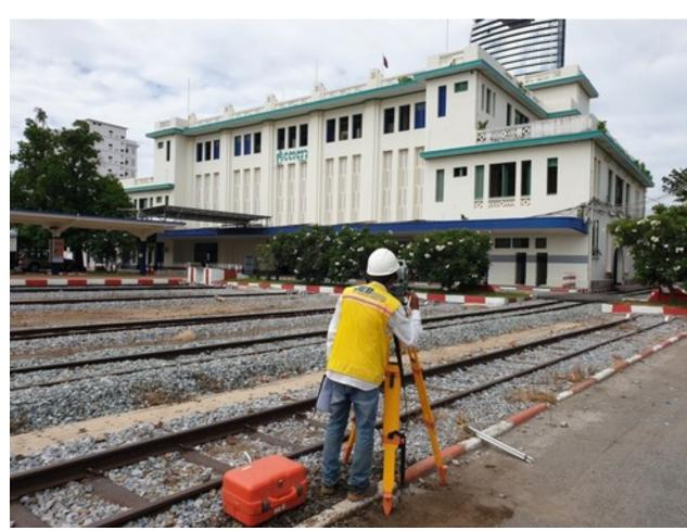
2019, JEB surveys & engineering provided an architectural and a non destructive structural survey work for Phnom Penh train station. We provided drawings with the exact building geometry and all the necessary documentation to conduct an up to date structural analysis.
